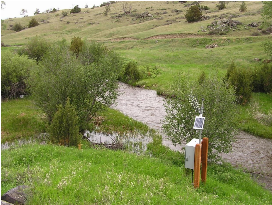
A U.S. Geological Survey streamgaging station on Willow Creek near Harrison, MT. Because of funding reductions, the DNRC is discontinuing seven streamgages that are cooperatively managed by the state and USGS. Credit: USGS
